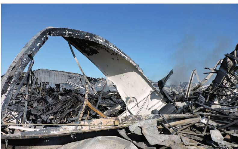
Shearer's Foods was virtually unrecognizable Feb. 23, 2022, following the explosion and fire Feb. 22. On Tuesday, March 8, a statement from the company said it is "exploring opportunities to relocate team members interested in working in our other plants" and has "provided a severance and benefits continuation package to recognize the effort and tenure that has gone into making the site successful over the past years."
