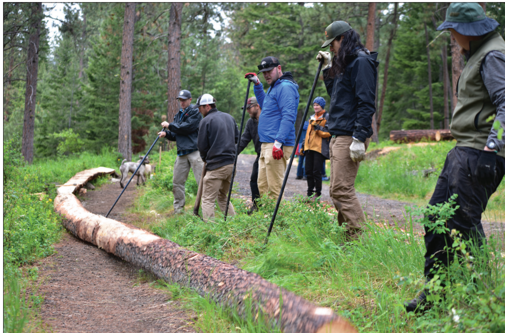
Volunteers at the Mount Emily Recreation Area's annual work day for nonmotorized trails prepare to install a "skinny" — a narrow pathway for mountain bikers to train on — from a split tree at the site's Skills Development Center Saturday, May 22, 2021. The skinnies help mountain bikers prepare to handle the 8- to 12-inch-wide trails at the recreation area.
