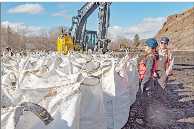
Ellen Morris Bishop/For the Wallowa County Chieftain Nez Perce Tribal Fisheries biologists Montana Pagano, left, and Kate Frenyea look at the “supersacks” of soil and gravel to construct temporary cofferdams in July 2021 when the side channels are connected to the Wallowa River.
