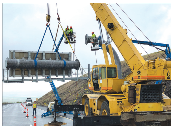
Crews installed one of the new message reader boards along the freeway as part of the two-year I-84: Snow Zone Safety Improvements Project. The project included about a dozen such signs between Pendleton and La Grande, along with new cameras, road sensors, lighting and other enhancements.
