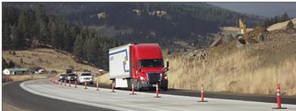
As part of the Ladd Canyon Freight Improvement project, a new third lane for east-bound trucks heading up Ladd Canyon grade east of La Grande was open for traffic in early November.
