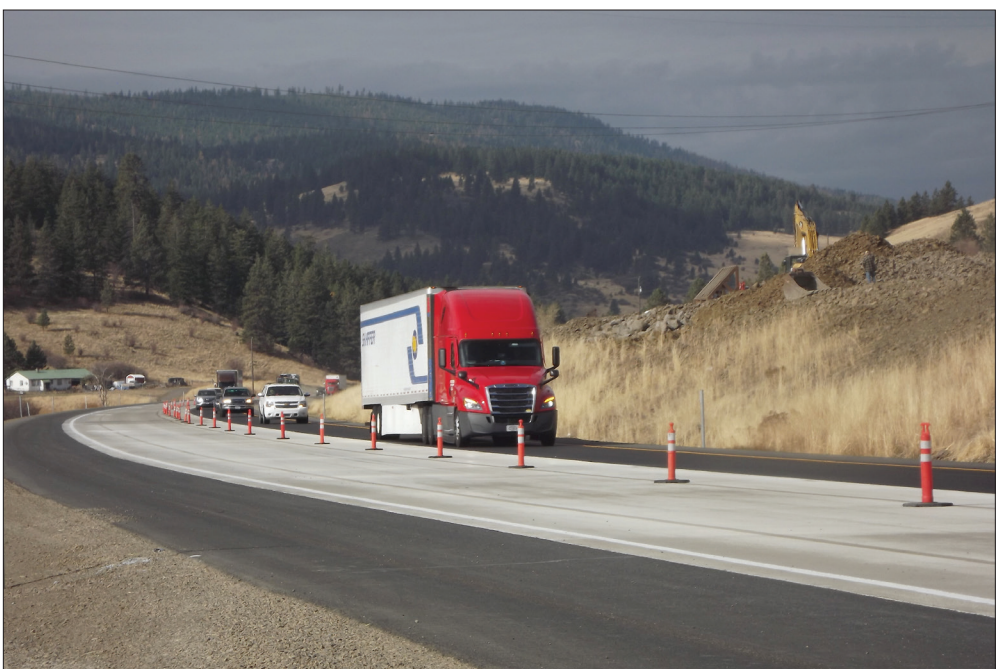
Dick Mason/The Observer Vehicles roll through the Ladd Canyon work zone Thursday, Nov. 5, 2020, on Interstate 84 south of La Grande. The Oregon Department of Transportation is finishing its improvements along the stretch of Ladd Canyon, including a new concrete lane for passenger vehicles.
