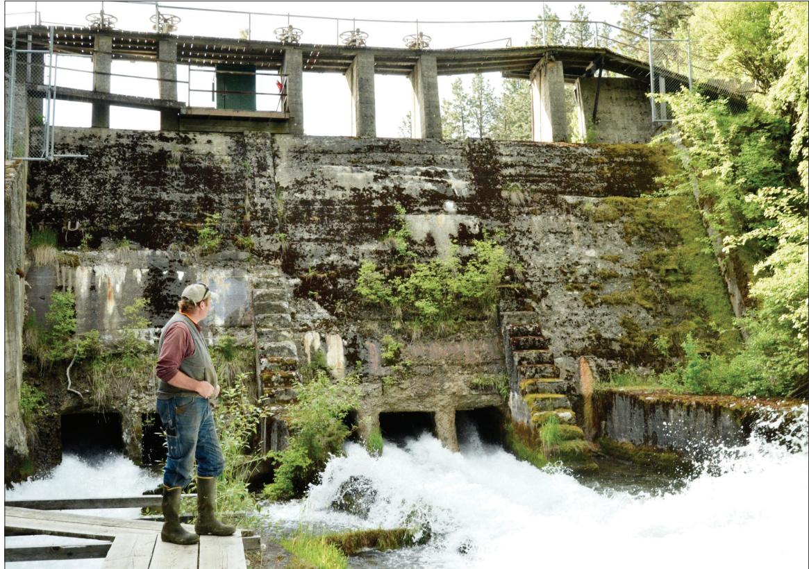
Blane Hayes, caretaker of the Wallowa Lake Dam for the Wallowa Lake Irrigation District, looks up at the dam Friday, June 12, as water from the lake flows through at about 400 cubic feet per second.
