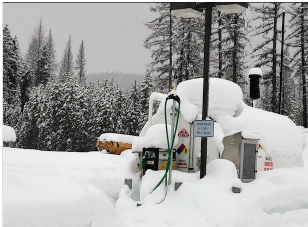
Snow covered everything at the ODOT Austin Maintenance station last winter.
