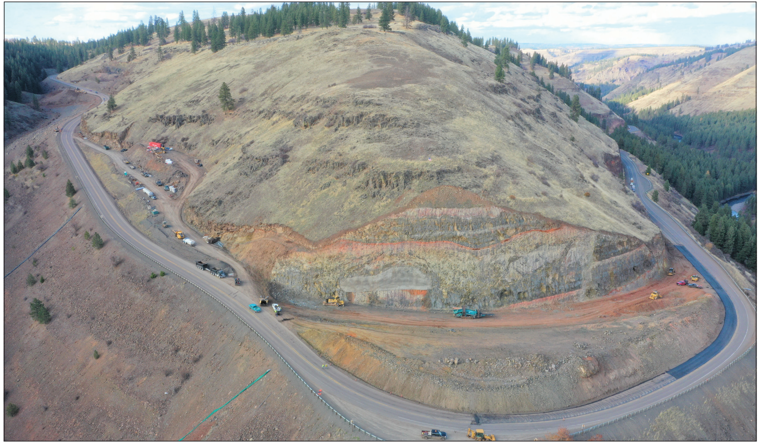
Work progresses on the OR 82 Minam Curve Project
