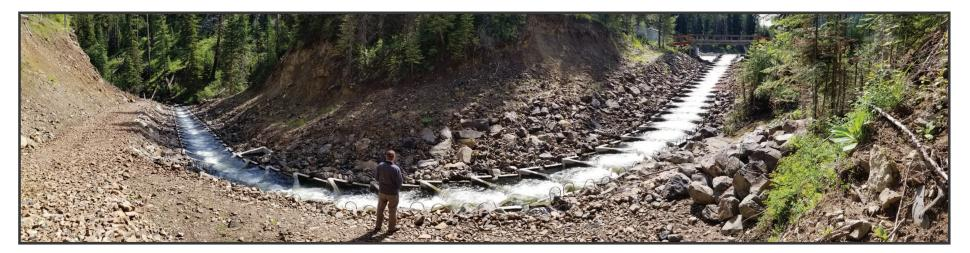
The Beaver Creek fishway allows access for steelhead, which were found spawning in Beaver Creek above the reservoir. These spawning grounds were previously inaccessible for more than 100 years (courtesy of Winston Morton).
