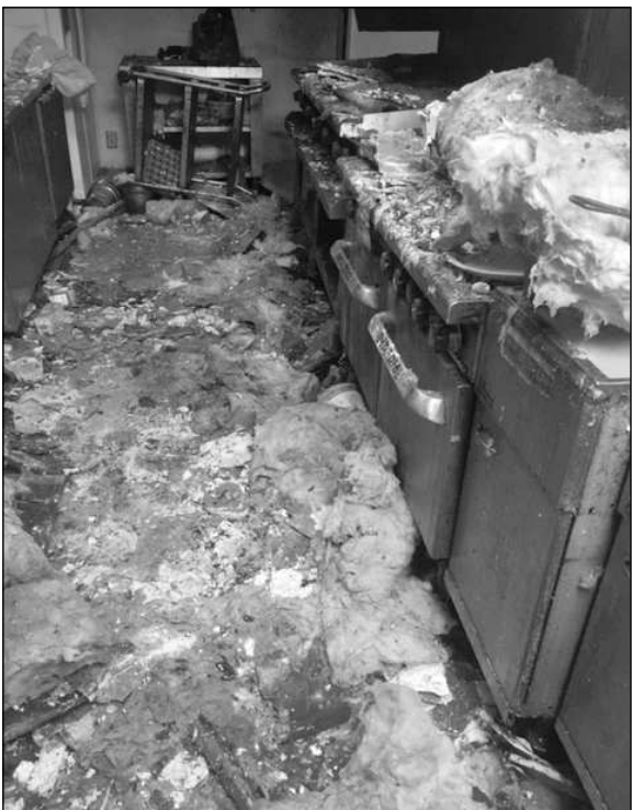
The fire's aftermath in the kitchen of Inland Cafe.
