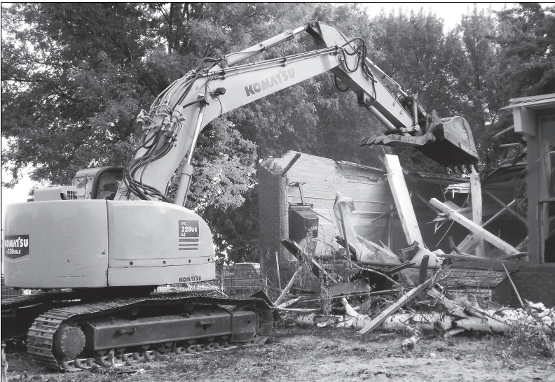
Funds from a bond Imbler School District voters passed in 2010 helped pay for the construction of a new elementary school, top, which opened in 2012. Demolition of the old Central Elementary School building, bottom, was completed in 2018.
