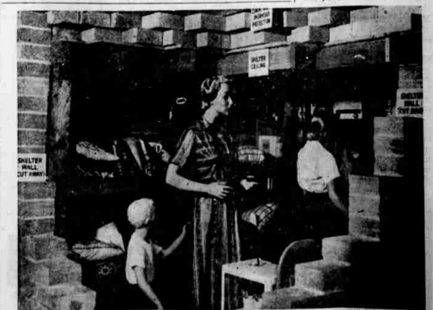
SURVIVED THE BLAST—These show window mannequins survived the blast and radiation effects of gigantic Nevada Proving Ground nuclear explosion when certain phase of the tests was based on A-bomb shelter protection. This particular shelter was made of concrete blocks and constructed in basement of model home located several thousand yards from point of detonation. Upper structure of house was badly damaged. The 8-inch solid concrete block walls would give the same fallout protection as 12 inches of earth. Note the food and other supplies stored in shelter.
