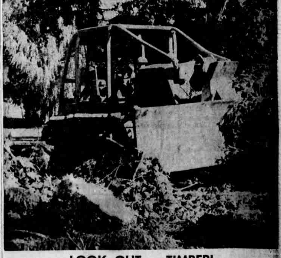
LOOK OUT... TIMBER! Joe Bekkedahl uses a bulldozer to knock down trees in front of Greenwood school. The crew's work was only routine until one of them spotted a large bee hive high up in one of the branches. Emergency measures brought the limb crashing to the ground. One crew member dashed to the hive and took care of the matter with a sauce pan of diesel oil. (Observer Photo)
