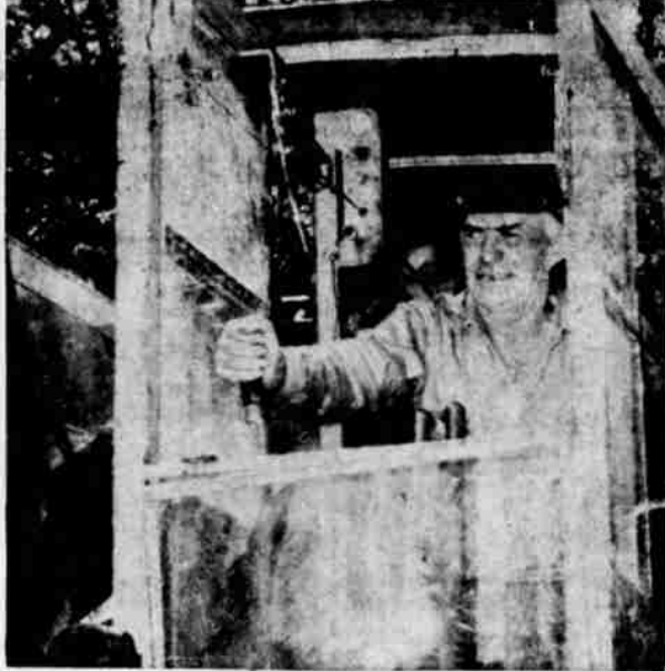
SHOVELING—Tom Perzell is working the shovel for the construction crew on the highway west of La Grande. The new highway will probably not take many miles off the trip to Pendleton but should eliminate many dangerous curves according to the State Highway Department. (Observer Photo)
