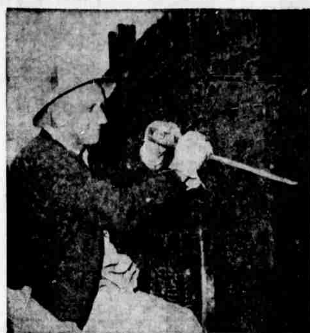
REPAIRING —Oscar Renas, above, is helping to repair the Grande—Ronde Apartments. Remas is working on the third floor which will be rebuilt.
