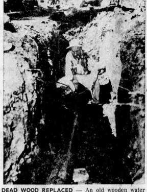
main, which leaked, near Oak and Spruce streets has been replaced by cast iron pipe as part of the city's program of replacing the old wood system. Earl MacDougal of the city water department is shown making a service connection just before the new pipe is covered. The old wood pipe was left in the ground disconnected.
