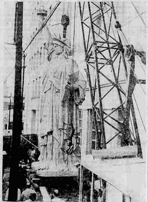
LIBERTY RISING—What at first glance looks like the Statue of Liberty in unfamiliar surroundings is actually a one-fifth-size replica of America's famous Lady. The 31-foot, 29,000-pound bronze statue is being hoisted to the top of the Liberty National Life Insurance Building in Birmingham, Ala., where its gas-fired torch will shed light 184 feet above the city. Like her big sister in New York Harbor, Miss Liberty was made in France.
