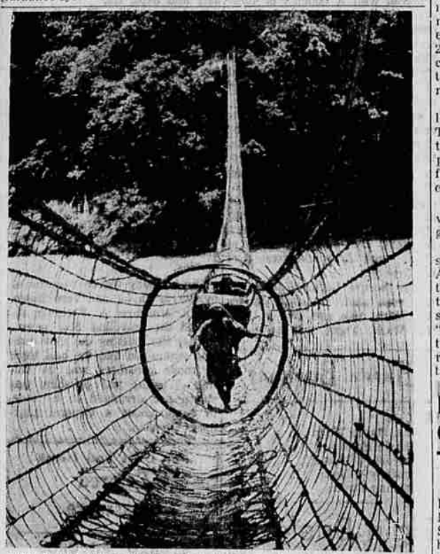
WALKING THE WEB—Though this looks like the work of a giant spider, it is actually an ages-old bridge form in Tibet. The two women are crossing a river in the Loyu area of Tibet on a cane-rope bridge.
