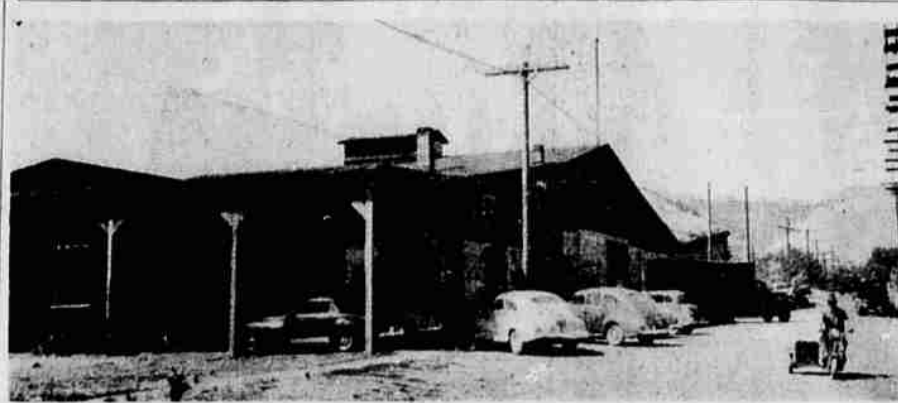
PAUL BUNYAN TRAILER COMPANY HOME at 1602 Cove avenue, which has been enlarged and modernized. The offices and parts department, formerly housed in the main building, have been moved into the new east wing.
