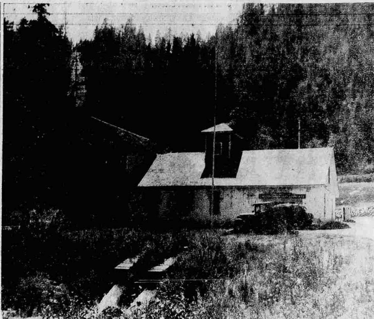
ROCK CREEK plant of the Eastern Oregon Light and Power company five miles and a half west of Haines in Baker county, at the foot of the Blue mountain range. Although the penstock is not shown in the picture it is a steel pipe 2,720 feet long and the Pelton water wheels are rated at 880 horse. The generators are rated at 450 KW, 2,300 volts each. The total head is 960 feet, one of the first high head plants in the northwest. The substations steps up the voltage to 23,000 volts for transmission lines extending to Union, Baker and Grant counties. The Rock Creek plant is the dispatching center for the system, it controls the loading of the plants, switching of lines and other details of the system operation.
