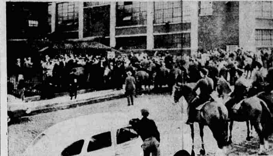
AFL OIL WORKERS PASS THROUGH CIO PICKET LINES—Cries of "strike breakers" and "scab" accompany 300 AFL building trades employees as they pass through CIO picket line at Standard Oil company refinery at Cleveland, O., under watchful eyes of police. AFL construction workers have been barred from working inside plant gates since CIO Oil Workers Union struck for 30-cent raise.
