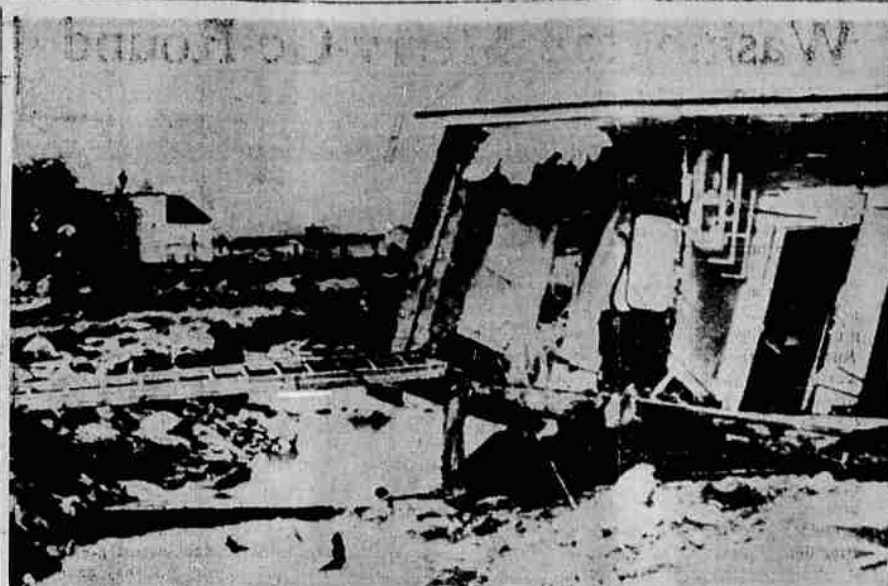
FLASH FLOODS SWEEP FOUR STATES —Rampaging Kinderhook creek, swollen to river size in cloudburst, swept Steventown, N. Y., home off its foundation and washed away Rutland & Chatham railroad bridge. Damage to highway and other property in Steventown was high and flash floods caused millions of dollars worth of damage in New York, New Jersey, Massachusetts and Pennsylvania.
