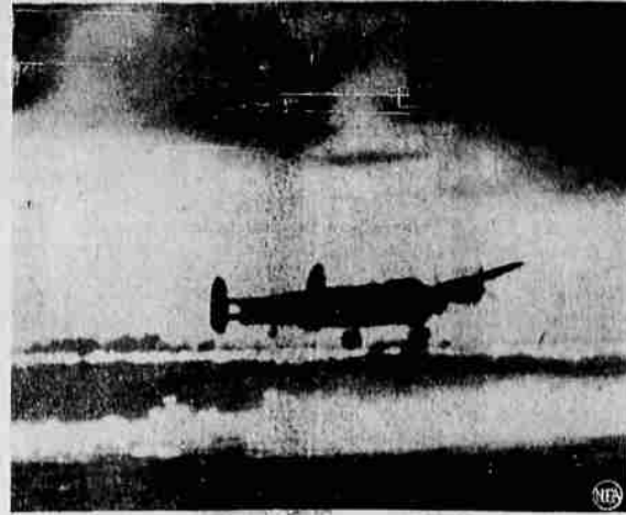
FOG-DISPERSING 'FIDO' IN ACTION—This first photo to be released on "Operation Fido" (Fog Investigation Dispersal Operations) shows how fog was artificially dispersed from RAF airfields by lines of burners on each side of main runways. In the picture, an RAF Lancaster is taking off, from clear-vision field, though fog hangs heavy up above.
