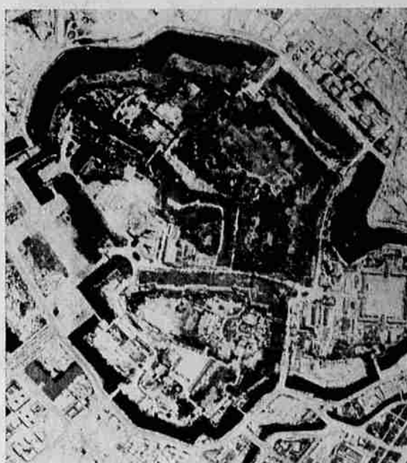
EMPEROR'S PALACE GROUNDS BOMBED—Numerous buildings within Emperor Hirohito's palace grounds as well as adjacent areas are burned out following two fire raids over Tokyo by more than 1,000 B-29s which dropped 8,500 tons of fire bombs. The emperor's palace is the dark circular area in center and bombed-out palace buildings are shown as light portion at bottom of area. Over 18 square miles of Tokyo were burned out in these two missions. 21st bomber command photo.
