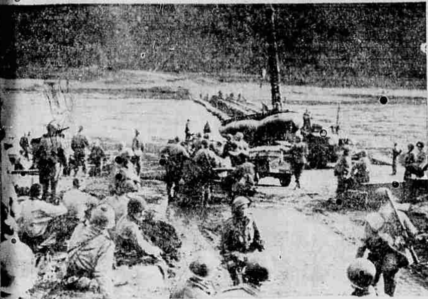
THIS IS HOW THEY DID IT—Third army engineers lay down a pontoon bridge across the Moselle river in a dress rehearsal for crossing of the Rhine which was made in conjunction with a crossing by three armies in a final push against Germany. This scene was duplicated for miles up the stream.
