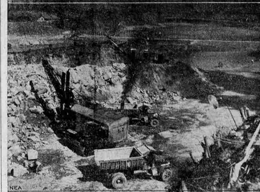
Scene of activity at the Bonneville dam and hydroelectric development project on the Columbia river, Oregon, where 1300 men are engaged in preliminary work harnessing the river. When completed the dam will raise water level of the river 82 feet, generate 105,000 horsepower and extend slack water navigation range some 100 miles above Portland, metropolis of the district.
