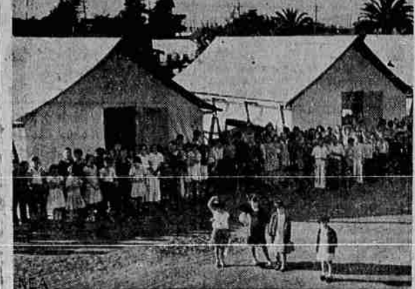
More than 140,000 Los Angeles schoolchildren have cloth schoolhouses now as the result of the Board of Education closing scores of buildings deemed unsafe in case of earthquakes. Here is one of the temporary schools and some of its pupils.
