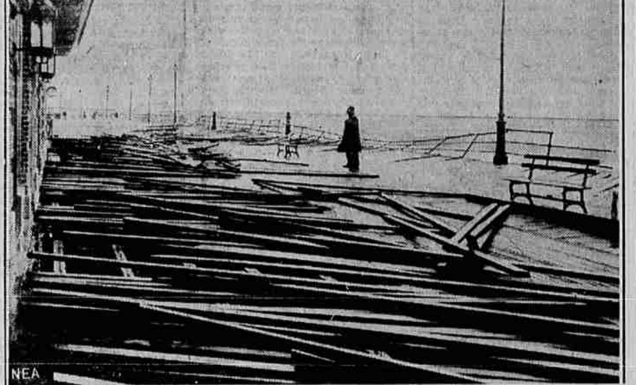
There was no strolling by honeymooners or vacationers on Atlantic City's well known boardwalk while the storm whipped at the famous New Jersey resort. Photo shows how the heavy planking was ripped up by the hurricane wave and wind.
