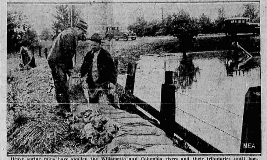
Heavy spring rains have swollen the Willamette and Columbia rivers and their tributaries until low-lying towns and farms have felt encroaching waters, and bridges have been washed out. This photo shows farmers working to strengthen a dike along the Columbia near Vancouver, Wash. Similar scenes are to be found in many rivers in Northern Washington today.
