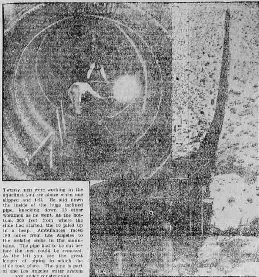
Twenty men were working in the aqueduct you see above when one slipped and fell. He slid down the inside of the huge inclined pipe, knocking down 15 other workmen as he went. At the bottom, 300 feet from where the slide had started, the 10 piled up in a heap. Ambulances raced 180 miles from Los Angeles to the isolated scene in the mountains. The pipe had to be cut before the men could be removed. At the left you see the great length of piping in which the slide took place. The pipe is part of the Los Angeles water system now under construction.
