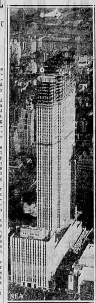
There it is — the biggest office building in the world! This picture was taken as the last girder was placed atop the central structure of the $25,000,000 Rockefeller Center development in New York. Seventy stories, and more than 800 feet, in height, it is not the tallest skyscraper but has the most office space.
