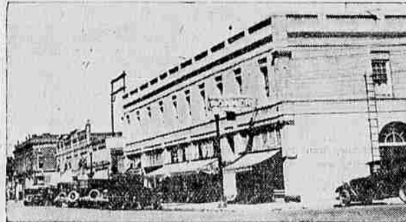
The Sommer Hotel, located at the corner of Depot street and Washington avenue, is a two-story structure covering approximately one-quarter of a block. The lower floors are rented to various business establishments while the entire upper floor consists of modern, well furnished rooms.
