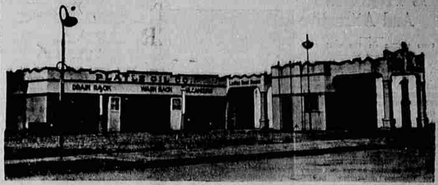
This large, completely equipped service station, owned by the Playle Oil company, and located at the corner of Adams avenue and Greenwood street, handles Texaco products, and specializes in prompt washing, greasing, and tire repair service.
