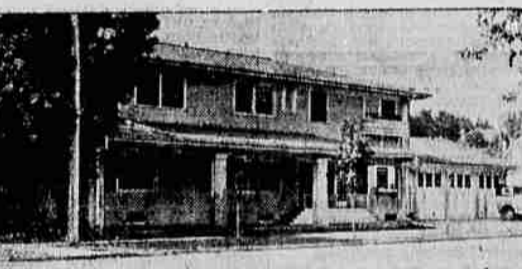
The Snodgrass & Zimmerman Mortuary is located at the corner of Fourth street and Pennsylvania avenue.
