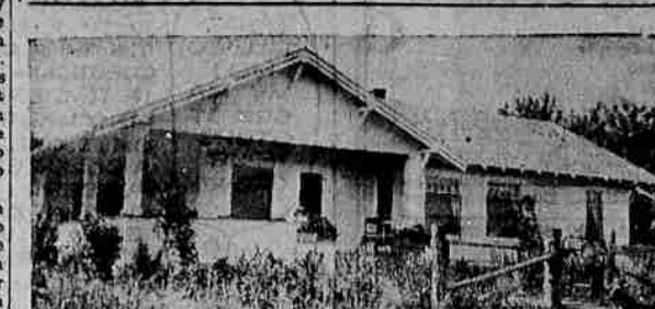
The above is a picture of the country home of F. G. Potratz, mid-way between Pleasant Grove and Summerville. The home is one of the attractive ones in that section of the valley. It was the former home of the late W. A. Baker and Mrs. Baker, prominent valley residents prior to their passing.
