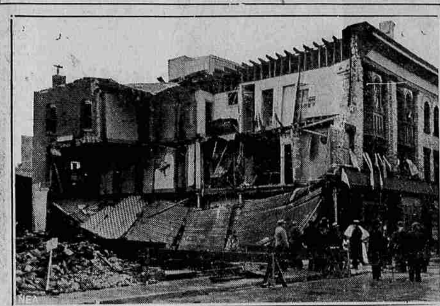
The force of the mysterious explosion which wrecked this three-story brick apartment building in Springfield, Mo., and claimed six lives, is graphically indicated in the above photograph, taken soon after the fatal blast. In addition to those killed, sixteen persons were injured when the explosion tore rooms apart on the second and third floors. Police investigated rumors that the structure was bombed.
