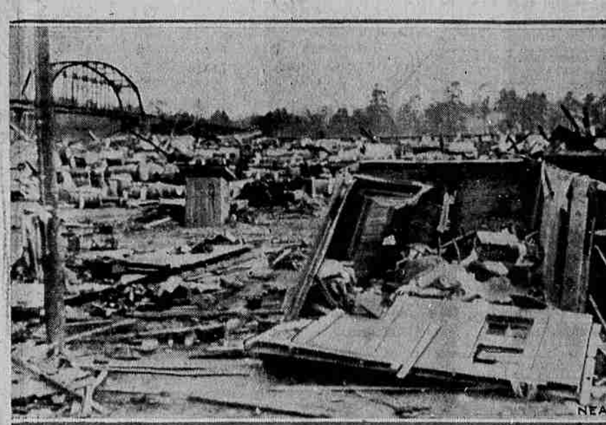
This first picture, rushed by plane from the storm area to Atlanta and transmitted by telephoto to San Francisco and thence north to the Observer, shows the havoc wrought by a tornado at Newport, Ala. It is typical of the appearance of a number of towns in the storm area, where nearly 400 persons were either killed or fatally injured.
