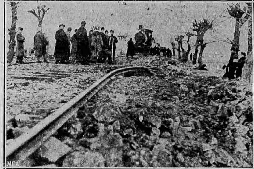
Japanese shells and aerial bombs found their mark. This picture, taken on a main line railroad near Kou-ping-tzu, Manchuria, shows how the tracks were ripped up by the heavy bombardment which preceded the fall of the city. Chinese workers are shown vainly trying to repair the damage before the advance of the Japanese forces while a train waits for clear passage.
