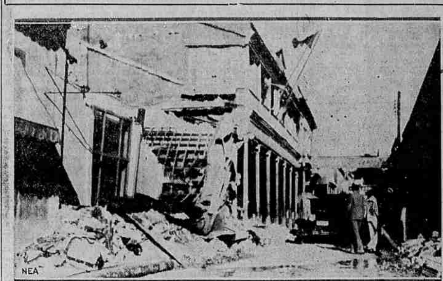
This picture, rushed from Santiago, shows some of the destruction wrought by the earthquake in that Cuban city Wednesday. Note how the building in the foreground has been wrecked. Picture rushed by plane from Cuba to Atlanta, Georgia, transmitted from there to NEA's San Francisco office and rushed to the Observer.
