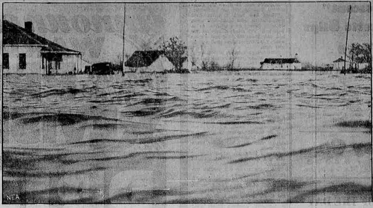
New levee breaks on Tallahatchie river flooded 50,000 acres and marooned 7500 persons in the Mississippi delta area below Memphis, Tenn. Flood conditions were described as the worst in history in the entire Tallahatchie basin. The photo here shows a street in Sharkey, Miss., just after a break in the levee had sent the swirling flood waters into the little town.
