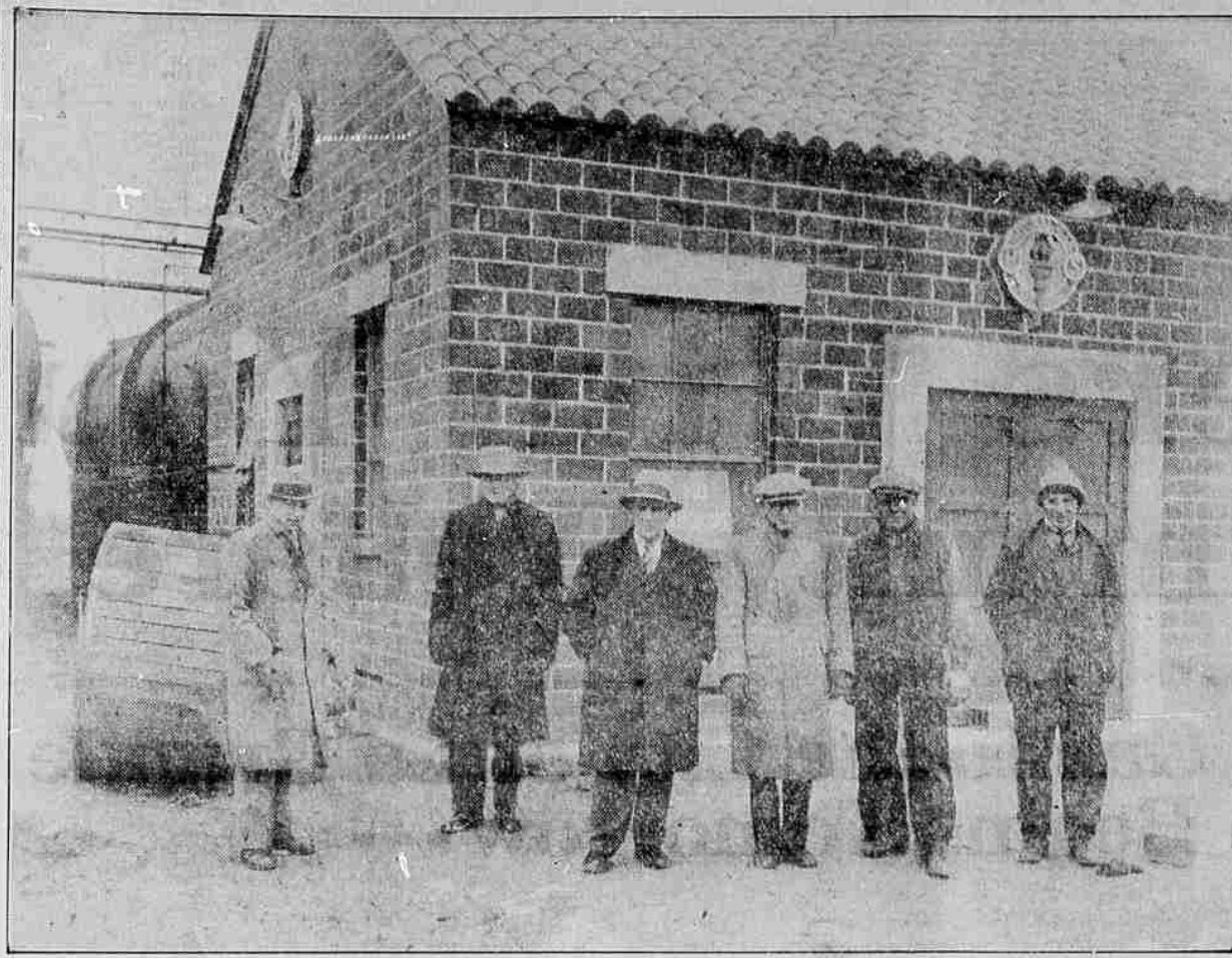
Photograph of Natural Gas Corporation of Oregon Building in La Grande which is now ready for operation. In addition to two employees of the company, the picture shows W. C. Crews, Charles Playle, William Condit and R. D. Scott, the latter being local representative of the company.
