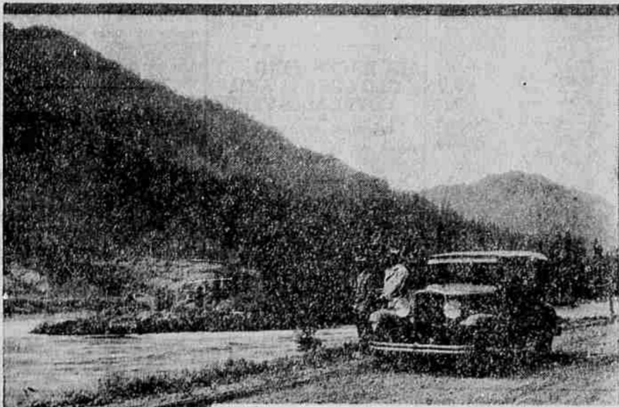
Local motorists who spend their vacations driving over the celebrated Columbia River Highway in Oregon will find the State of Washington is constructing a new roadway on the north bank of the famed Columbia River paralleling the former route. Photograph shows a Durant 6-14 sedan on the North Bank with its party gazing across the Columbia into Oregon.
