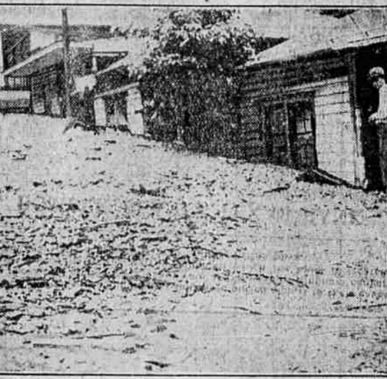
Many houses in Bingham, Utah, were buried almost to their eaves by rocks and mud when a heavy rain at the head of Bingham canyon sent a flood down the narrow gulch in which the town is located. Four years ago a snowslide took 37 lives in the town.
