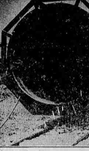
Prof. Georges Claude, French scientist, beside the giant steel tube which he built in an effort to harness the gulf stream and convert its waters into electrical energy. The tube which was 3,905 feet long and cost more than $1,000,000 collapsed and was lost as it was being lowered into the ocean near Havana, Cuba.
