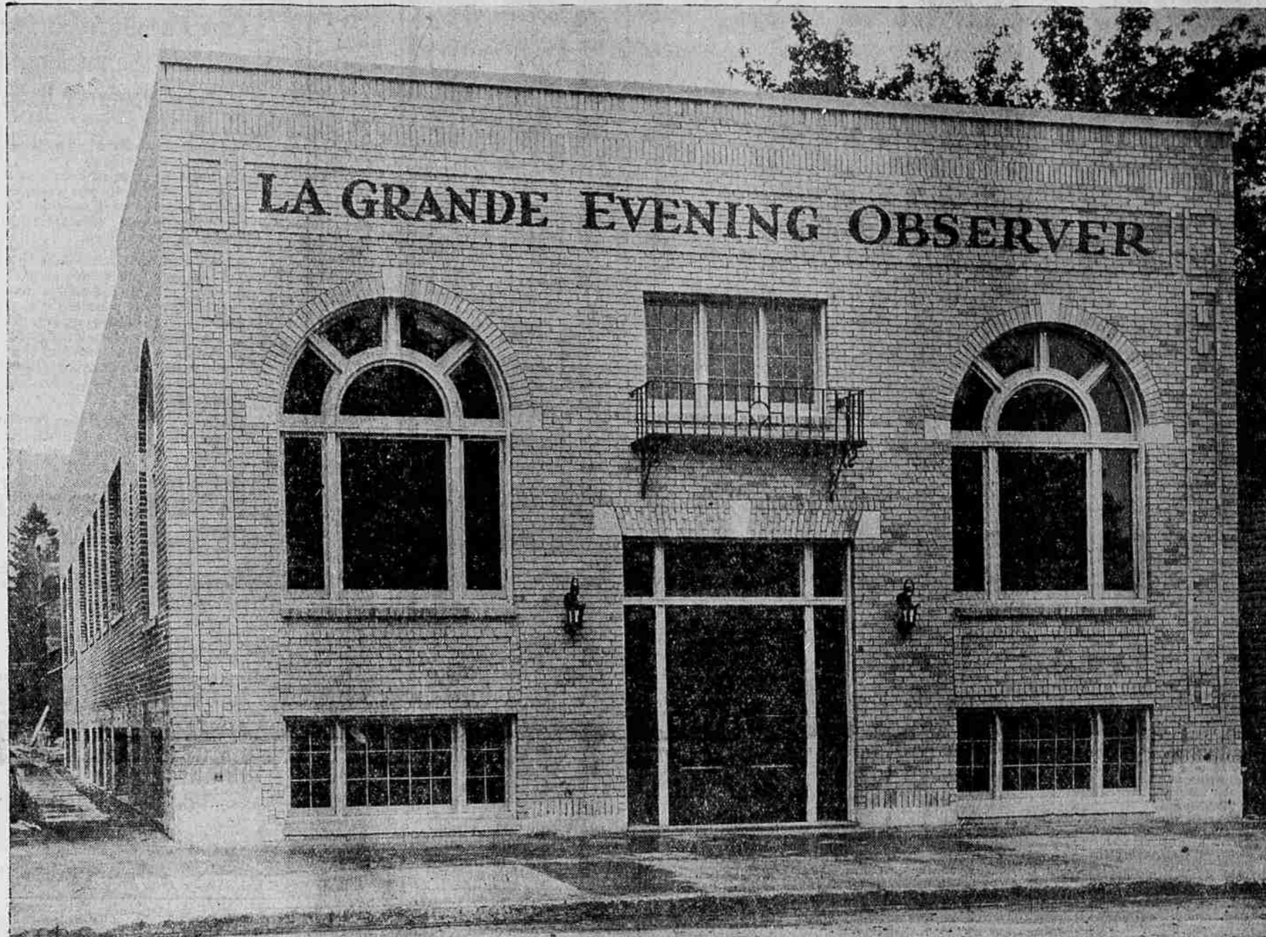
Front View Of The New Observer Building Facing Elm Street
