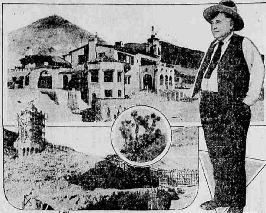
"Death Valley Scotty" (right) will have everything from a radio station to a six-foot hog fence around the desert palace (above) now building. There even will be a campanile with a carillon (below). In the circle is a Joshua tree, a type of vegetation on the place.
