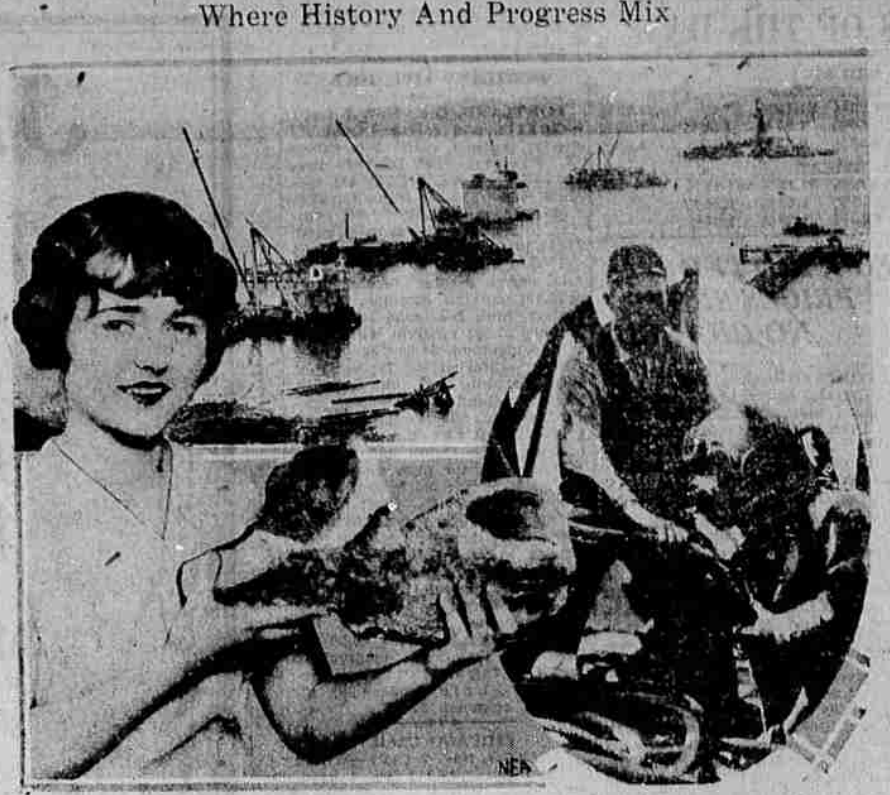
While doing preliminary excavation on the new S. P. railway bridge, which is to span Sulbut bay from Sulbut point to Army point, engineers have examined large quantities of fossils and mastodontic fragments...
