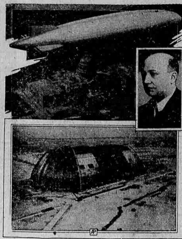
An artist's conception (above) of the navy's next dirigible, the ZIN-4, floating over the capitol at Washington. The ship, on which construction will begin soon, was designed by Dr. Karl Arnstein (inset). Below is a new hangar at the dirigible port maintained by the Goodyear-Zeppelin company at Akron, Ohio.
