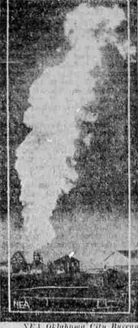
NEA Oklahoma City Bureau Here's a scene that proves bringing in a gas well isn't always profitable. This one, near Oklahoma City caught fire as it blew in, and caused a loss of approximately $50,000 to its owners before the blaze was ex- tinguished by "shots" of 200 pounds of nitroglycerine.
