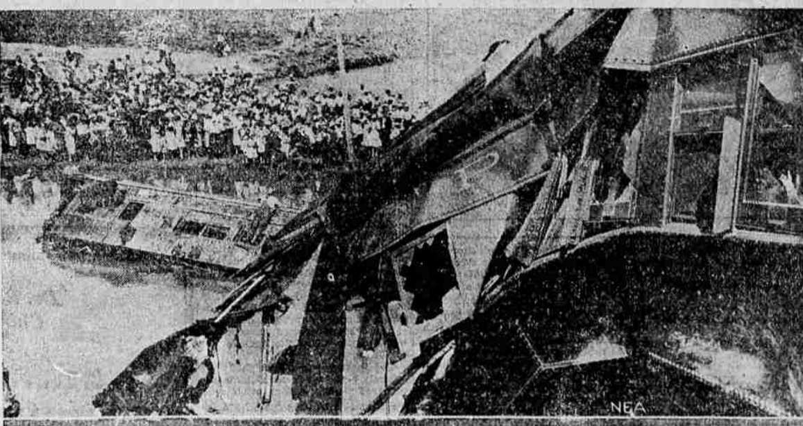
Here are some of the scenes near Stratton, Colo., Thursday when the crack Eastern Express of the Rock Island Railway crashed through a flood-weakened bridge carrying several coaches and their sleeping occupants into the torrential creek, with death by nine, and injury for others. Photos show various views of the havoc, including a glimpe directly across the creek, with the bare supports showing where the rails and span tore away.
